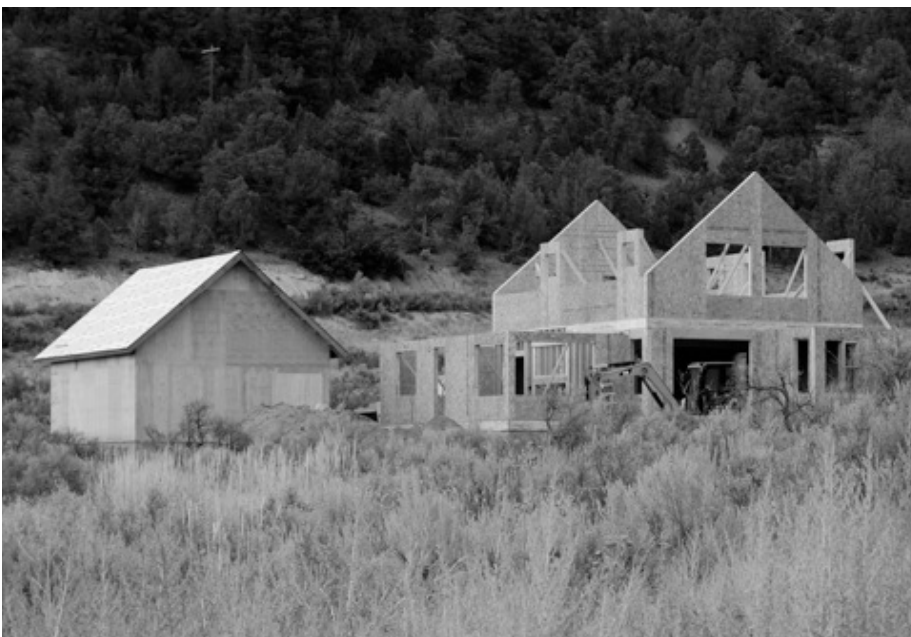
Construction Photo, Residence
